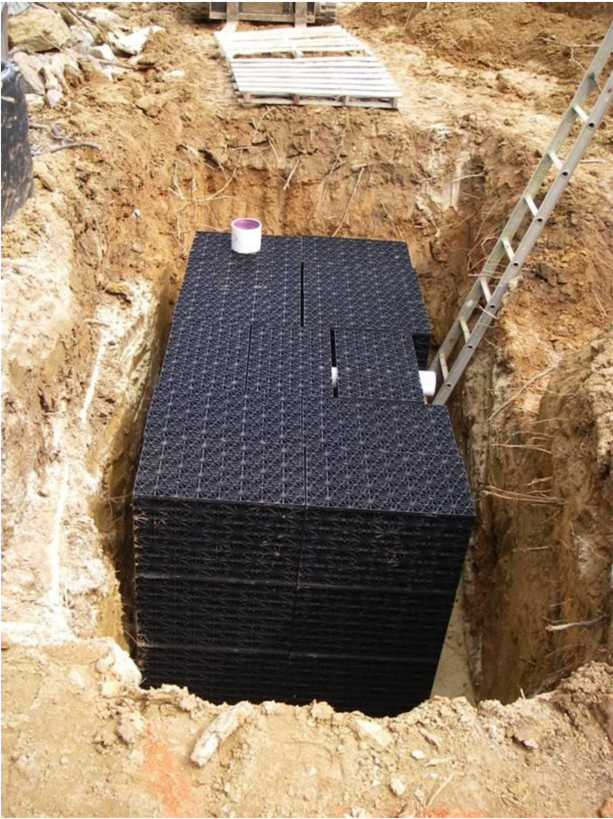
A drywell in place.
