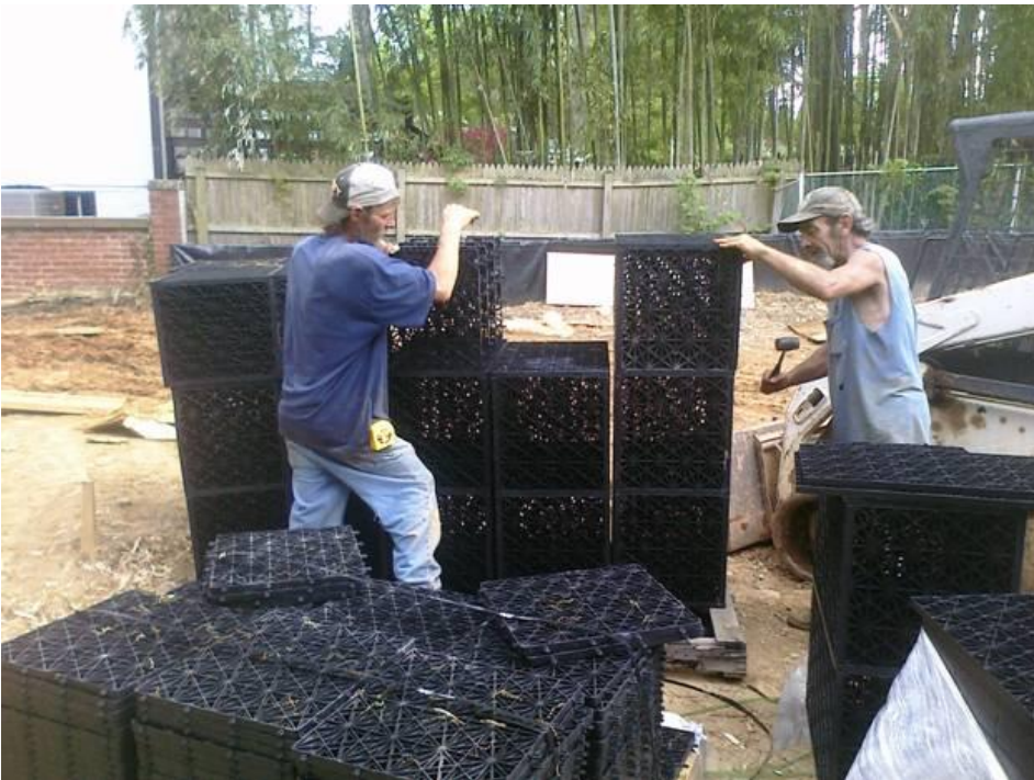
Drywell being set up.
