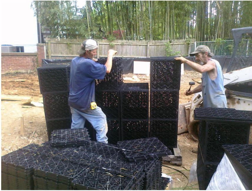
Assembling a rain tank on a homebuilding site. Scale of the tank and room needed is a reason sites are clear-cut rather than leaving the ability to spare a tree or two on-site during construction.
