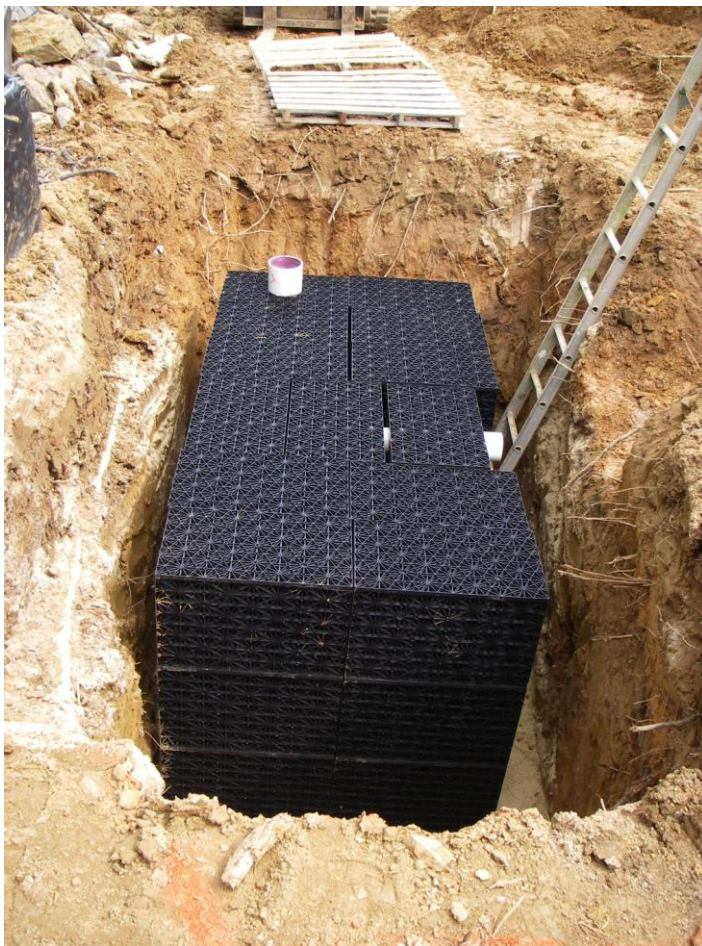
Assembling a rain tank on a homebuilding site. Scale of the tank and room needed is a reason sites are clear-cut rather than leaving the ability to spare a tree or two on-site during construction.
