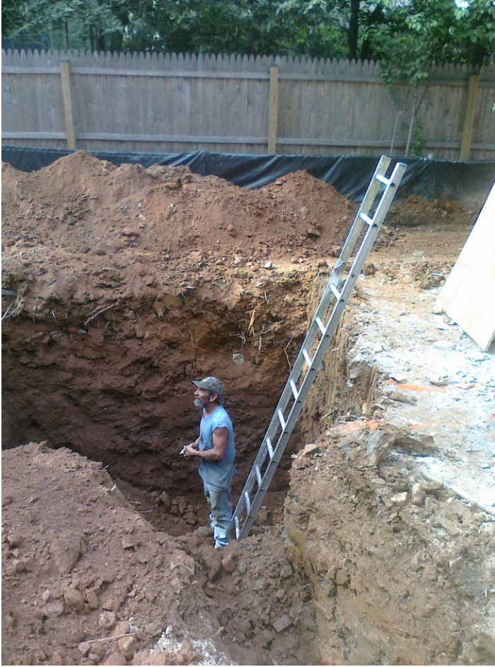
Examples of raintank install. This site requires 7 of these for house roof downspouts and driveway and must be 20' apart and 20' from house. It definitely is a destructive and ravaging process to get these in and really impossible to save anything around them or on the way to them.
